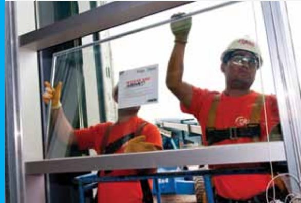
Sage glass, being installed at the Siemens - US Nacelle Facility in Hutchinson, Kan., is designed for energy efficiency.
